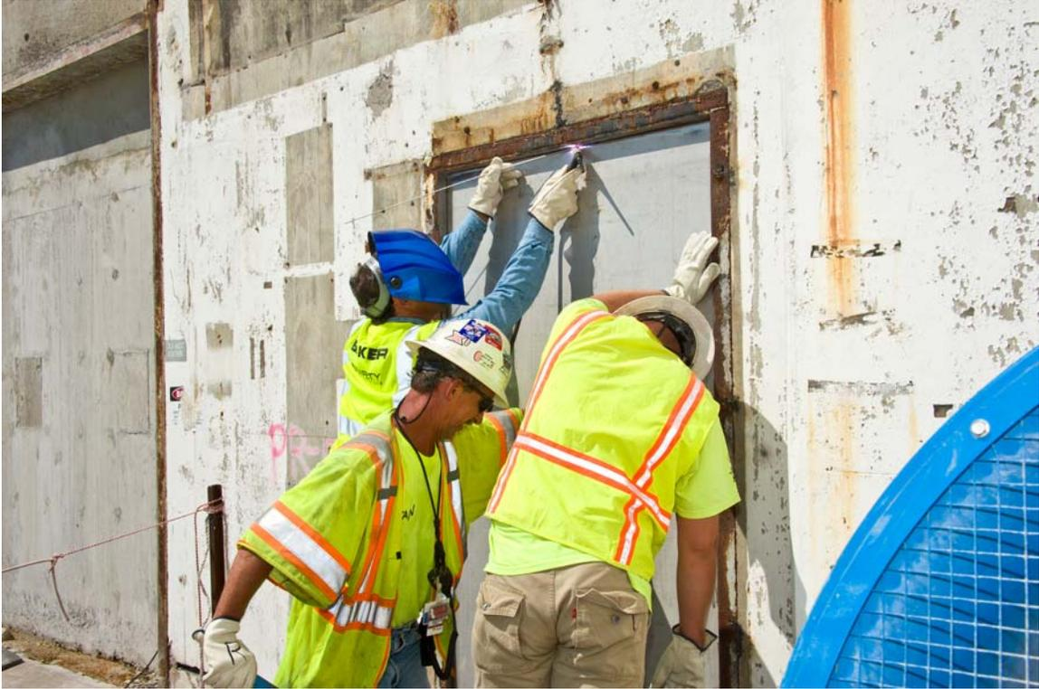
From left, Baker Concrete's Charles Powell, Archie Jarrell, and Michael Carter weld shut the last opening to the P Reactor 105-P building. Baker performed the in situ grouting of the below-grade areas.
