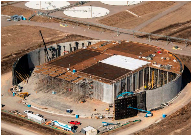
Saltstone Disposal Unit 6 at the halfway point in construction.
