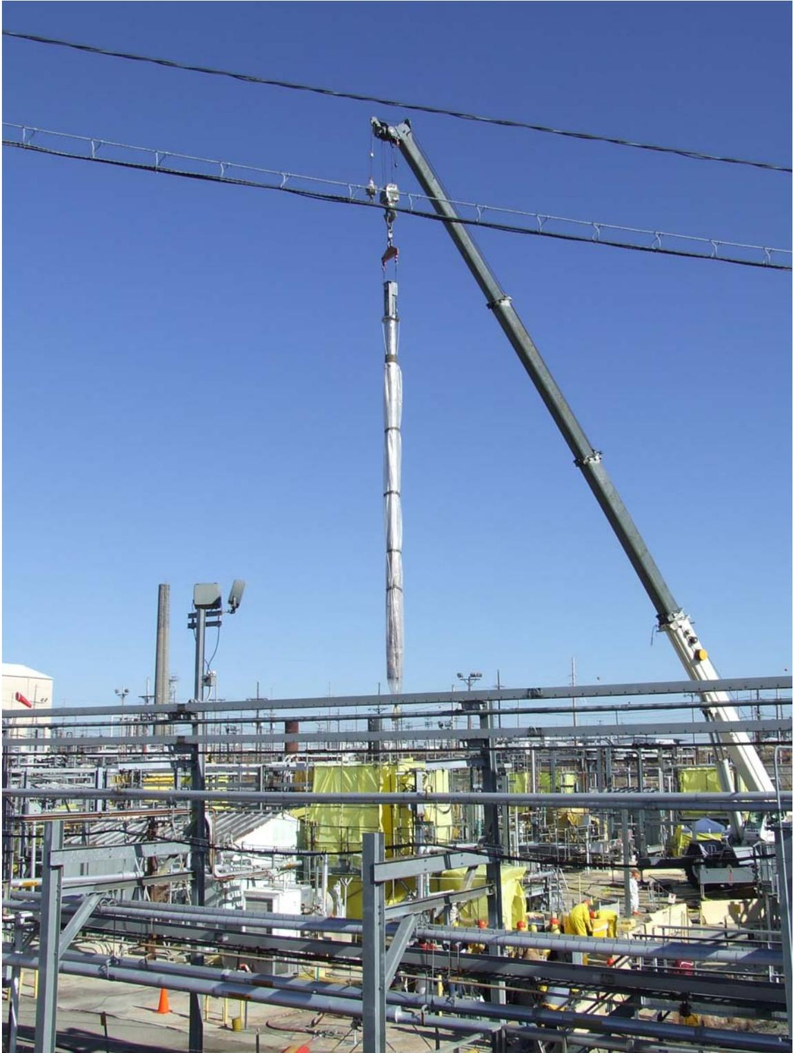
SRS workers remove 50 foot submersible pump from waste Tank 5 during completion of tank operational closure.
