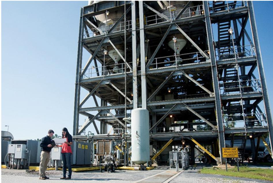
**Cutline:** Savannah River Remediation engineers Jay McCrary and Connie Yung work in front of the silos at the Saltstone Production Facility, where decontaminated salt solution is mixed with a cement-like grout for safe and permanent storage in Environmental Management’s Saltstone Disposal Units.
